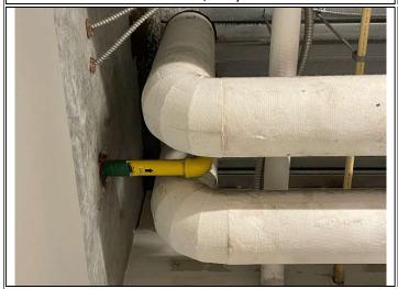
Photo 15: HM-N: Pipe Elbow Wrap, White
