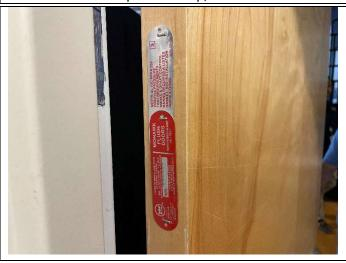
Photo 16: HM-O: Fire-rated Door Insulation, Red Label with Silver Lettering
